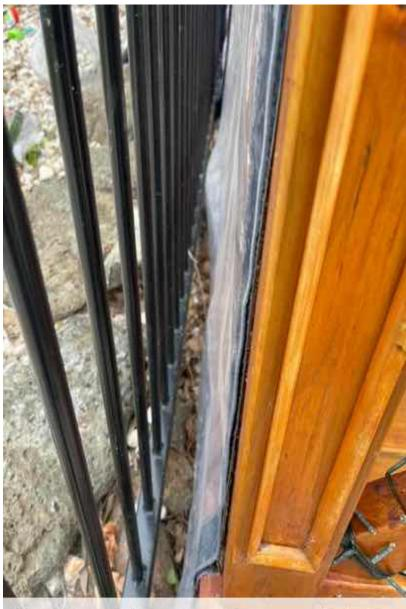
Screen needs to be secured permanently to the timber structure
